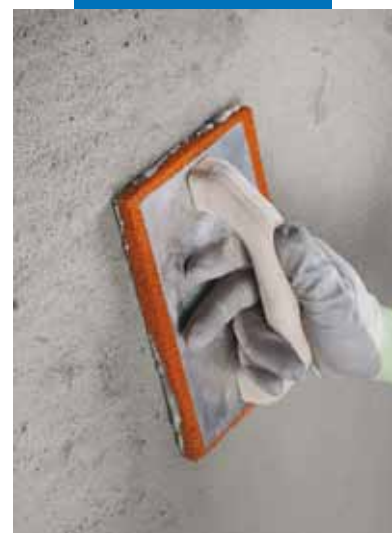
Tamping Planitop Smooth & Repair
