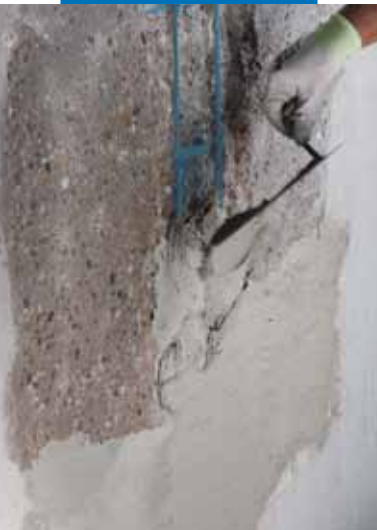
Application of Planitop Smooth & Repair by trowel
